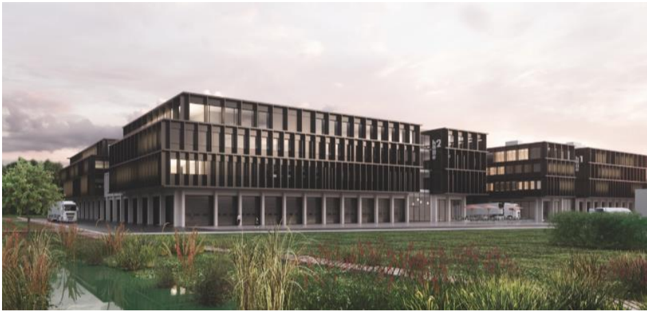
The new PULSE production and research buildings near Lausanne (image: © Architram et JBMN).
