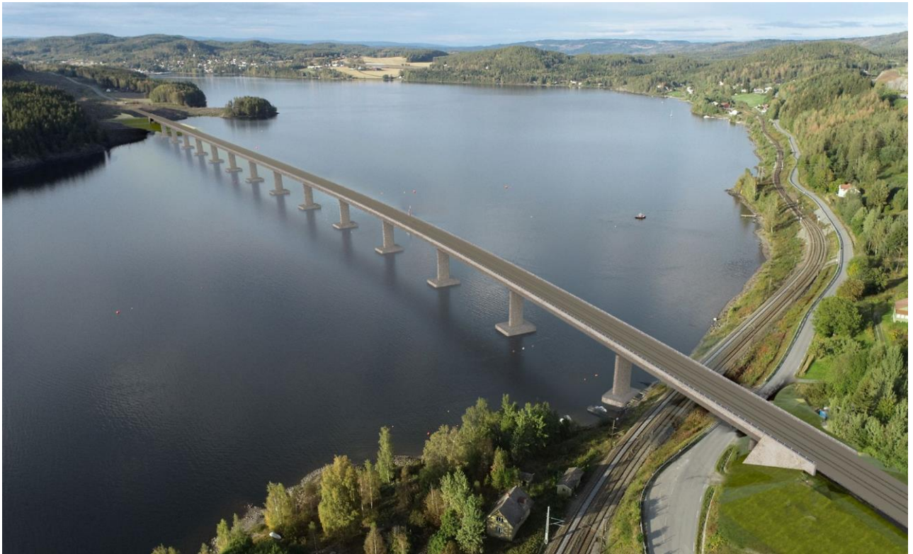
Tangenvika bridge: Fully digital model-based design and execution (image: ©Implenia/Norconsult).
