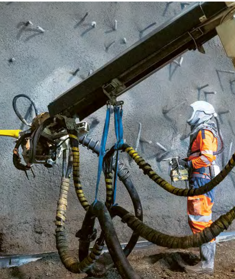
↑ Concrete is sprayed following installation of a centring frame
