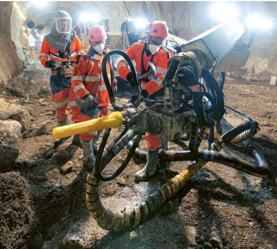
↑ Maintenance on the concrete spraying robot that applies the concrete made in the cement mixers.
