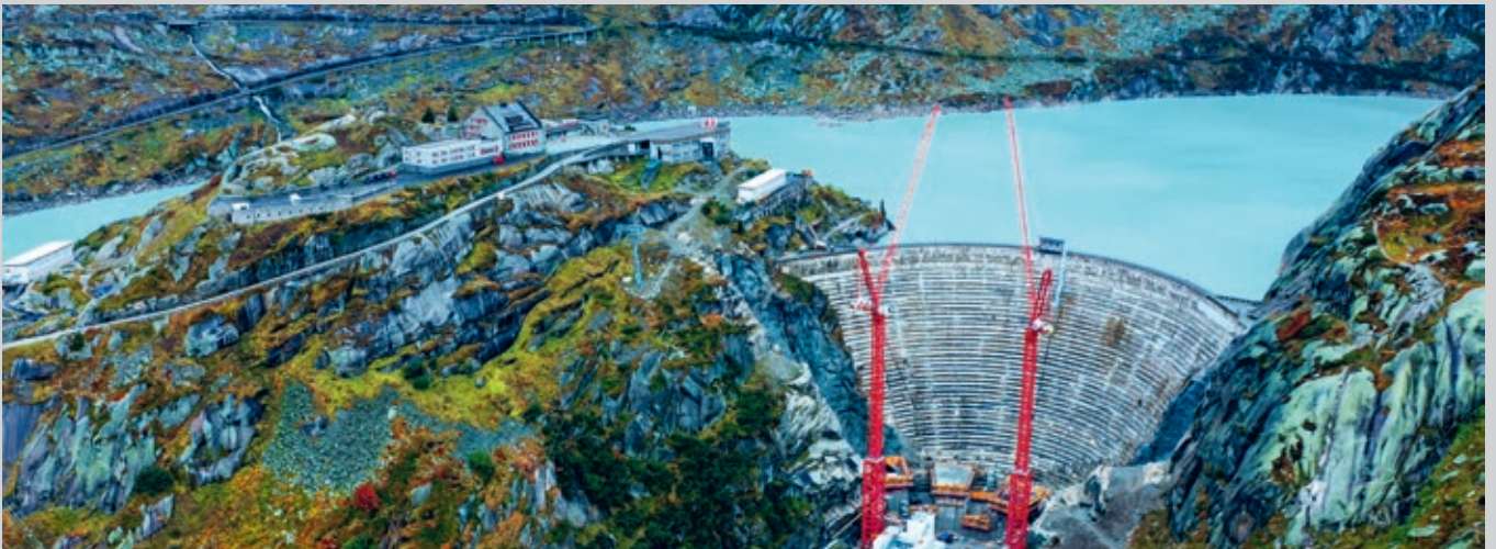
↑ Spitalamm: We are constructing a new replacement dam in front of the existing dam, at a height of 2,000 metres above sea level
